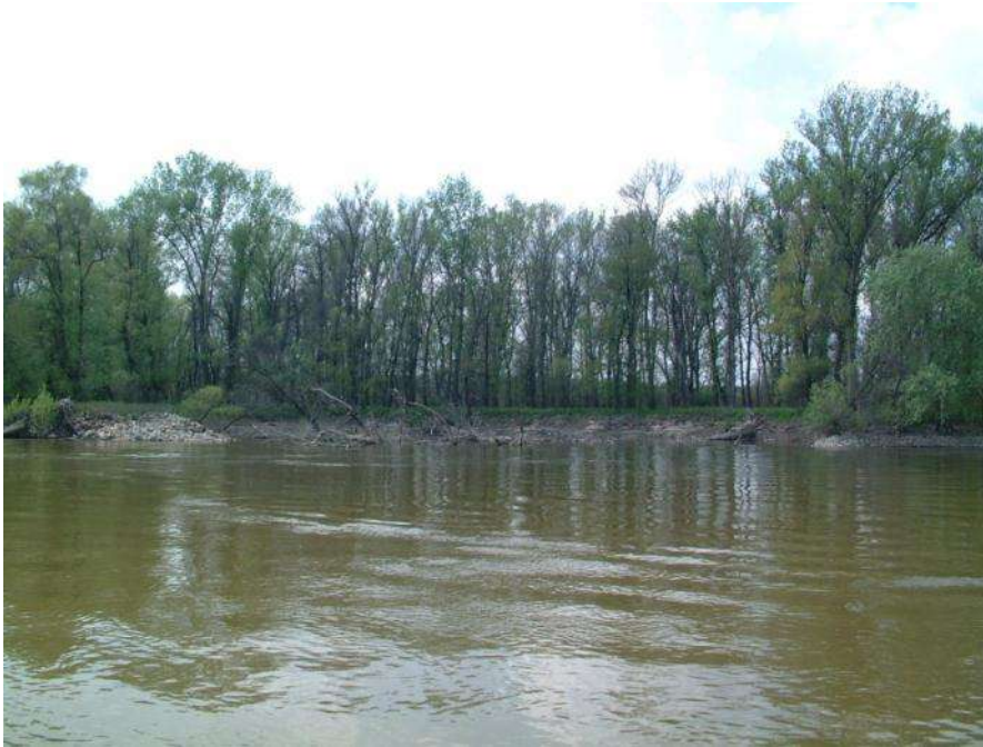
Figure 20: Collapsed bank revetment with radial pool development (© Ulrich Schwarz, FLUVIUS).
