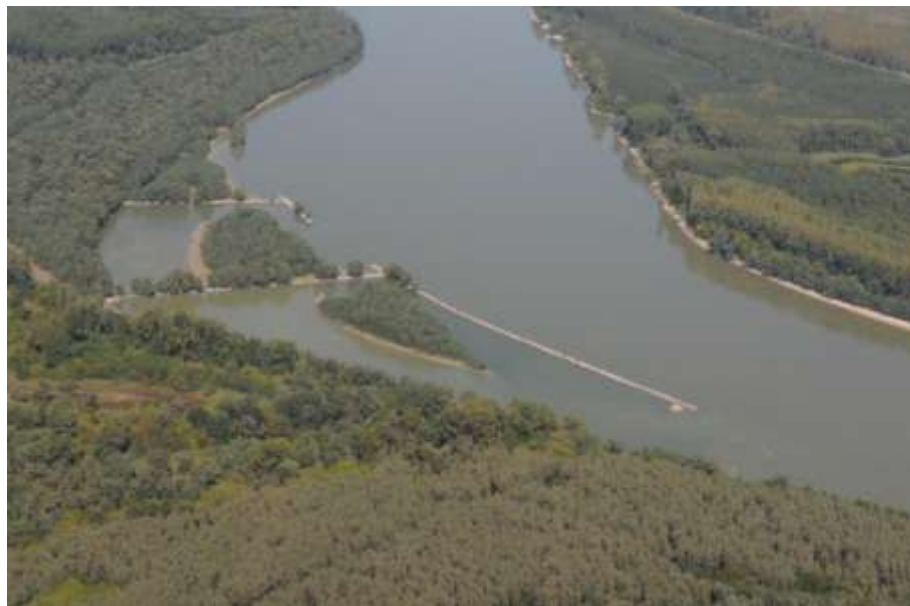
Figure 23: Reflectors (rip-rap guiding wall) (© Darko Grlica).
